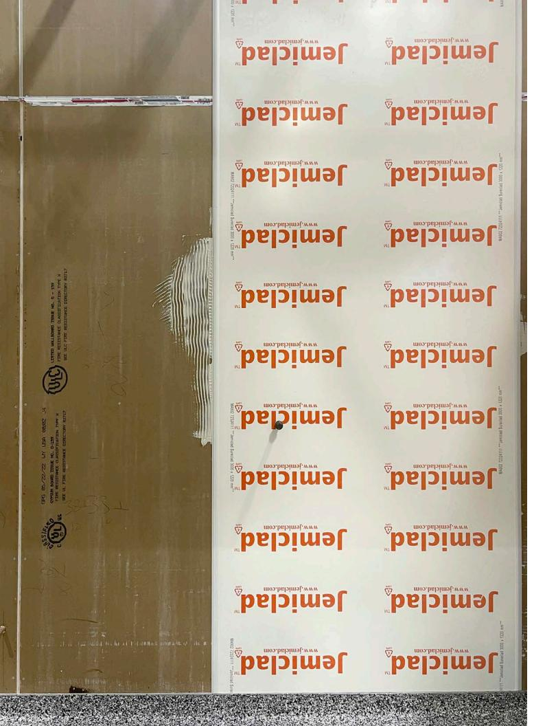
WELDED WALL PROTECTION AND INTEGRAL FLOORING COVE.
